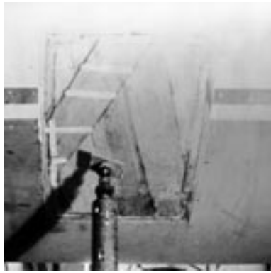
Figure 6-18 Bond the second layer in the opposite diagonal to the first layer.
