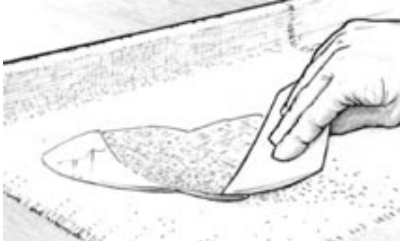
Figure 3-15 Spread the epoxy from the centre of the fabric toward the edges with a plastic squeegee or a roller.
