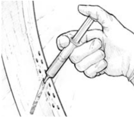
Figure 4-4 Inject resin/hardener mixture into holes until the damaged wood absorbs all it can.
