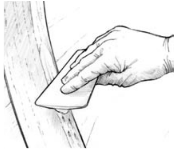
Figure 4-5 Fill the remaining voids with fairing compound.
