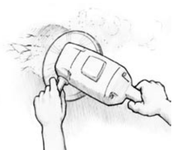
Figure 2-3 Grind out an area of many closely spaced or deep cracks with a disc grinder.
