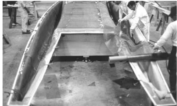
Figure 4-5 Breather material (bubble-type) is positioned over the release fabric after a manifold is in place.
