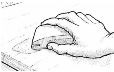
Figure 23 Sand cured fairing compound to desired contour.
