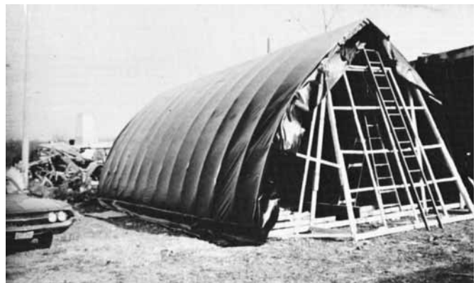
Figure 8-17 Plastic covering stretched over framework.
