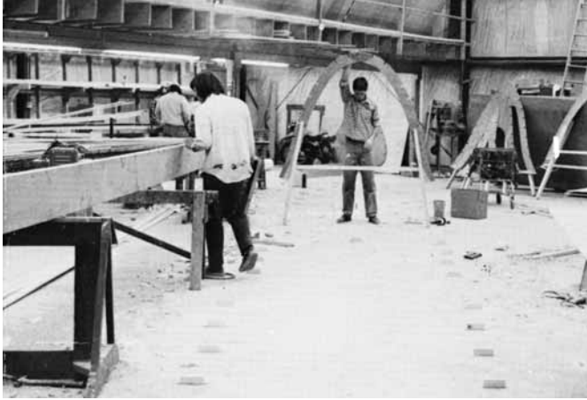
Figure 18-4 Setting up the first frame.
