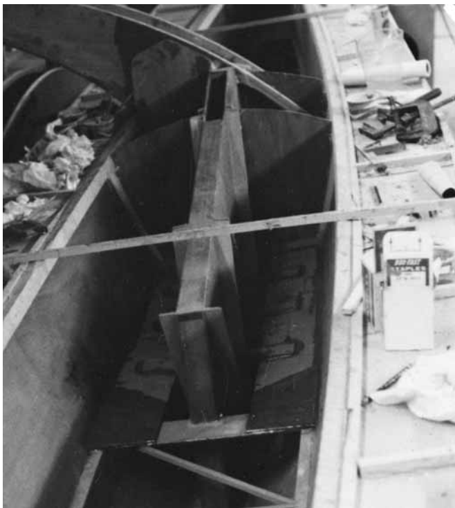
Figure 25-19 Structural members are installed in a 30' trimaran outrigger. One of the crossbeam arms and the centerboard case are braced and secured with the bulkheads and sub-level stringers in the foreground.
