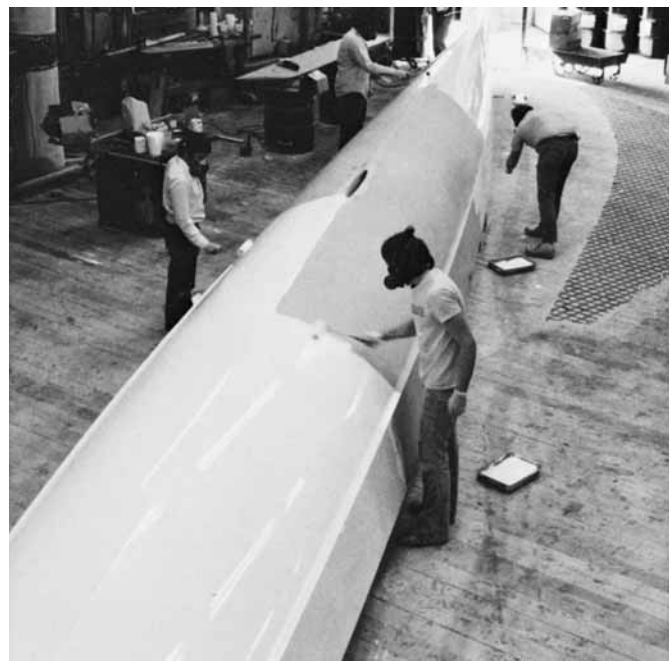
Figure 15-6 Rolling on two-part linear polyurethane paint.
