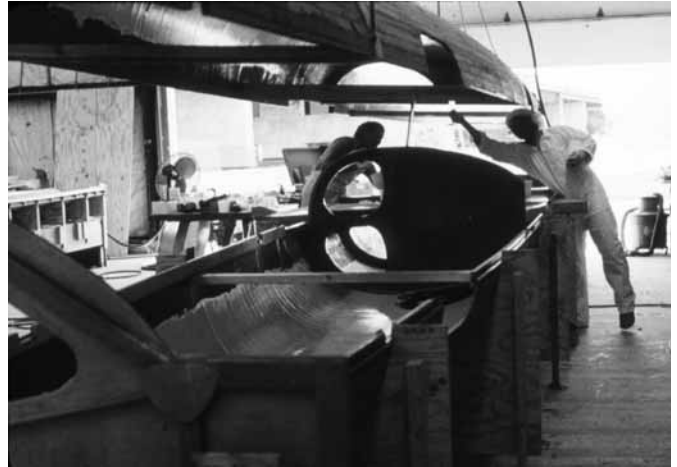
Figure 2-3 A bulkhead in position in the main hull of the Formula 40 trimaran Adrenalin .
