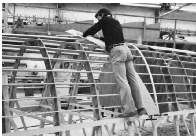
Figure 22-1 Rogue Wave's main hull set-up with stringers installed and ready for planking.
