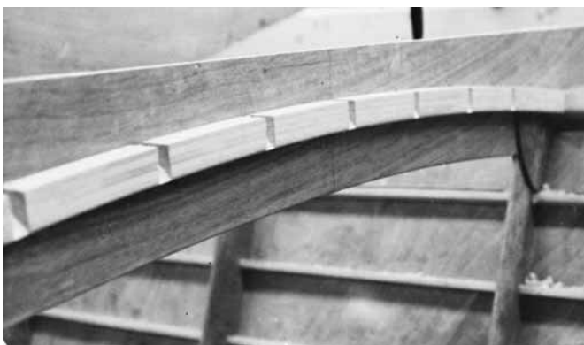
Figure 27-8 Triangular notches were cut into a laminated beam before it was bonded to the plywood frame. Longitudinal deck stringers were then easy to fit into the notches.
