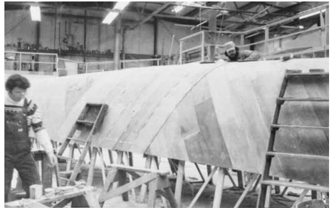
Figure 21-18 Installing a second layer of planking.
