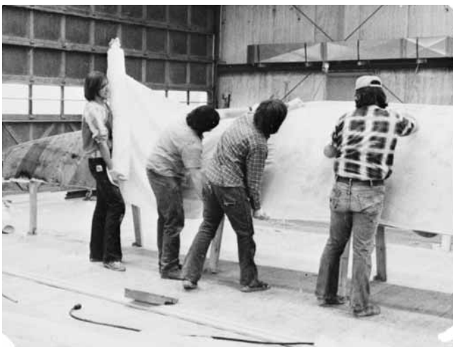
Figure 13-3 Applying polypropylene cloth to a 45' outrigger hull using the wet method.
