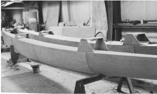
Figure 25-27 Construction on outriggers for a 35' trimaran. These hulls will now be coated and fiberglassed. See Chapters 13 and 15.
