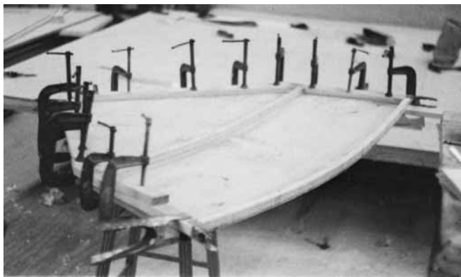
Figure 17-8 Building a laminated transom with cheek pieces.
