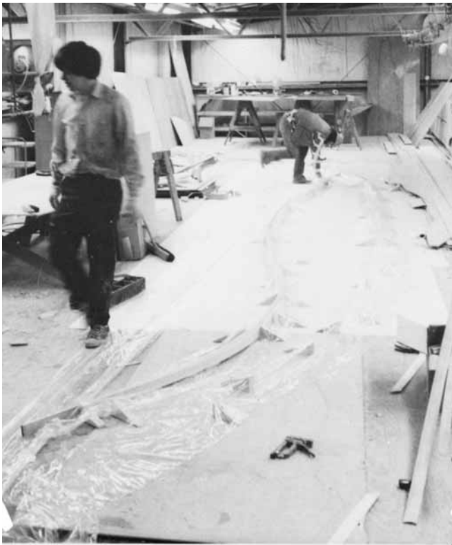
Figure 11-2 Laminating a long structural member for trimaran crossbeam using cleats secured to the lofting floor.
