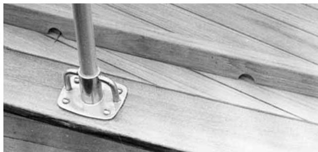
Figure 27-28 The intersection of the teak deck, a mahogany covering board, and cedar topsides on Golden Dazy . All three types of wood are no thicker than \frac{5}{32} " (4mm) and laminated in place with temporary staples. Note the teak toerail with limber holes.
