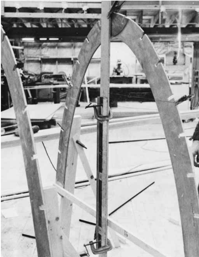
Figure 18-7 A straightedge clamped at centerline of frame.
