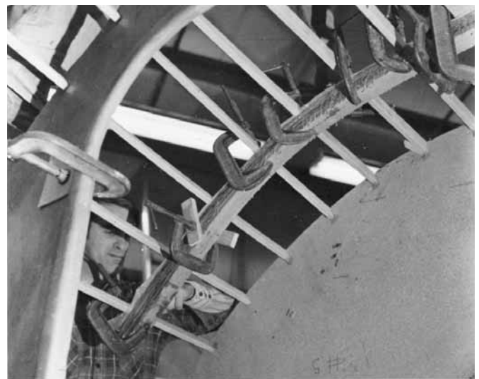
Figure 11-4 Laminating floor timbers using stringers as the form.
