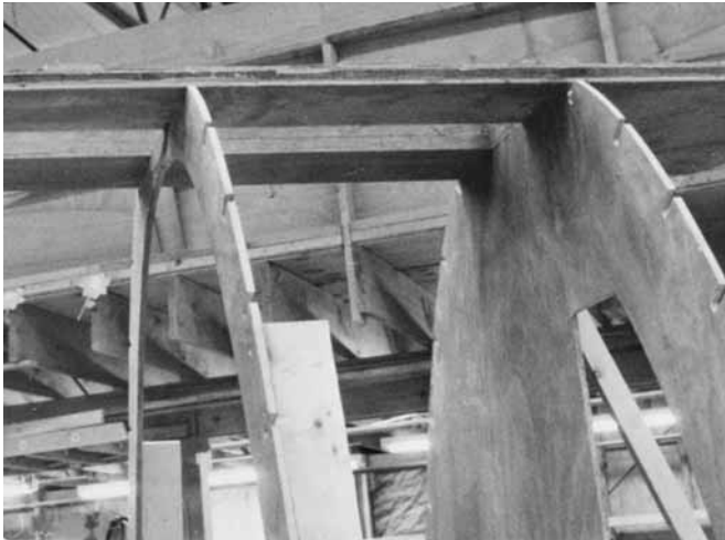
Figure 19-6 The laminated keel for Rogue Wave bonded to frames. The keel is ready to be faired. The frame crossing the centerboard slot will remain uncut through the planking process to prevent any distortion of the keel from stresses created during planking. The centerboard case was installed after the boat was turned over because, in this case, it was taller than the set-up allowed.
