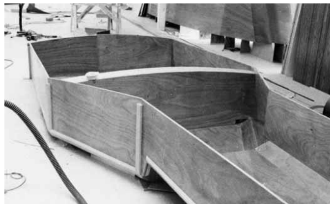
Figure 27-12 A cockpit assembly constructed outside the hull.
