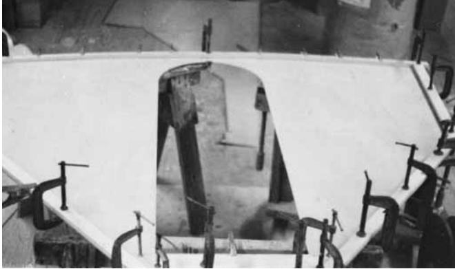
Figure 17-7 Bonding cheek pieces to a permanent bulkhead.
