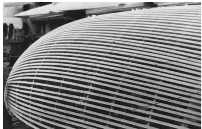
Figure 21-2 A ribband mold for a ½-ton racer showing alignment markings for various veneer layers.
