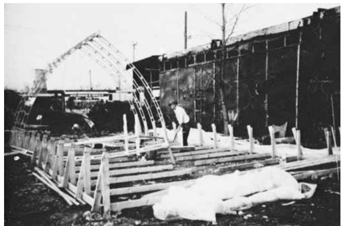
Figure 8-14 Assembling arches for a temporary shelter.
