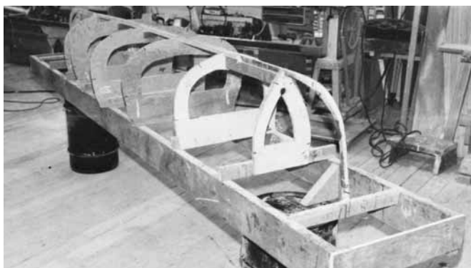
Figure 18-1 The strongback and mold frames for a small canoe. Note that it's often a good idea to raise a small strongback off the floor to a convenient working height.
