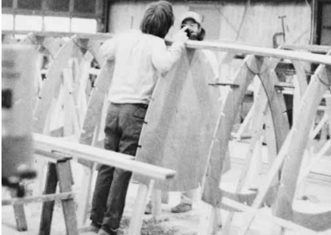
Figure 27-1 Web frames and deck beams in a set-up.
