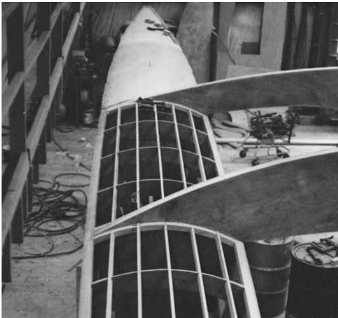
Figure 27-2 The same deck beams with stringers in place, ready for decking.
