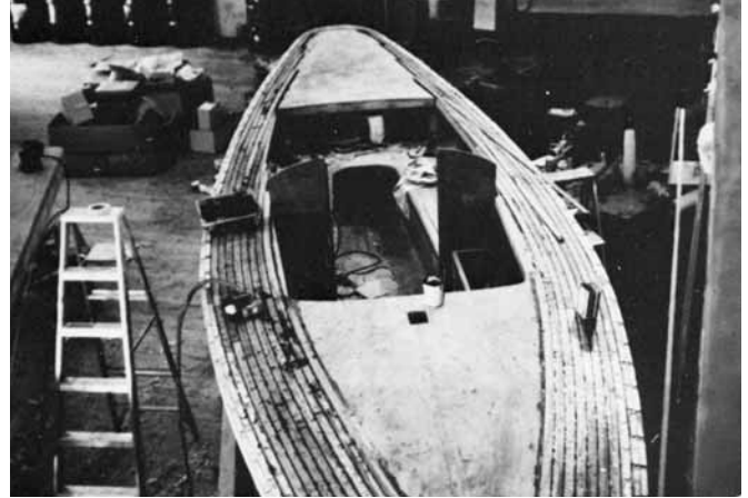
Figure 27-33 Installing teak planking parallel to the sheer, beginning along the outer sheer line and progressing toward the center of the boat. This is a sprung deck.
