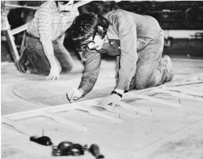
Figure 17-3 Transferring deck camber for a bulkhead from lofting to plywood stock using a batten and holders.
