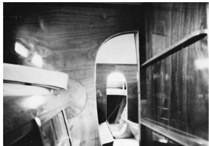
Figure 26-14 An opening in a structural bulkhead on Rogue Wave . The daggerboard trunk to the right is bonded to this bulkhead.
