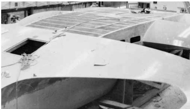
Figure 27-17 The foredeck and beam fairings on Rogue Wave are plywood over stringers. The cabin areas are sandwich construction using resin-coated paper honeycomb core.
