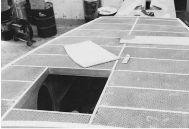
Figure 27-20 The aft deck on Rogue Wave with a 3" (75mm) thick honeycomb core between plywood panels.
