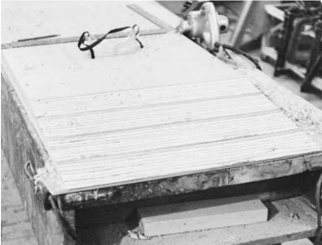
Figure 12-13 Cutting scarf bevels on stacked panels.
