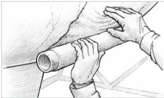
Figure 3 Unroll the fiberglass onto the surface with one hand—spread out wrinkles and press the fabric against the surface with the other.
