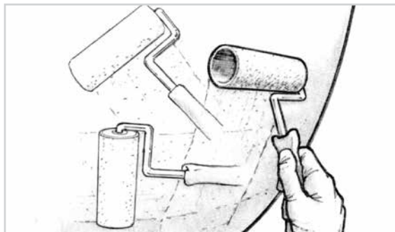
Figure 15-1 Using a foam roller, apply the epoxy and spread it into a thin even film.
