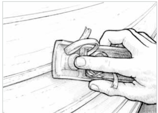
Figure 5-5 Use a plane to remove the excess spline and a sander to fair the surface after the epoxy has cured.
