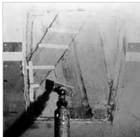
Figure 5-18 Bond the second layer in the opposite diagonal to the first layer.
