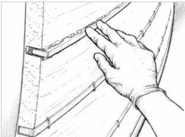
Figure 5-4 Push the wet-out spline into the seam.
