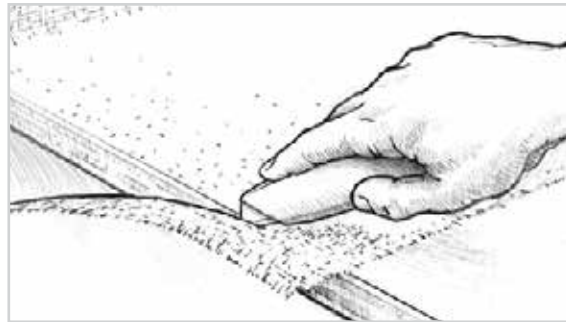
Figure 8-19 Trim excess cloth after the epoxy has begun to gel using a sharp utility knife.
