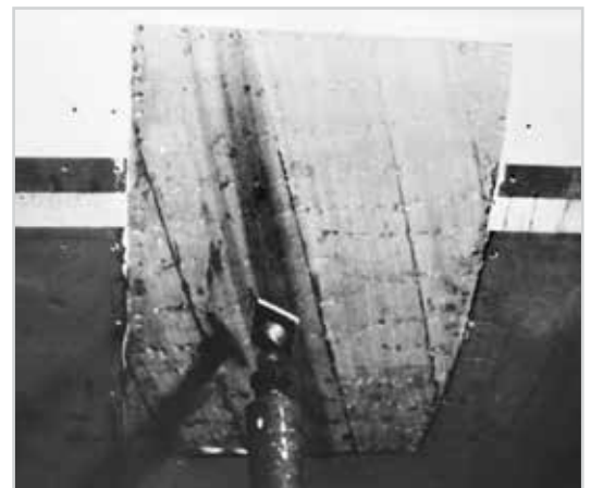
Figure 5-19 Continue until all the layers are completed, matching the skin thickness.
