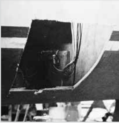
Figure 5-15 Remove the damaged section.
